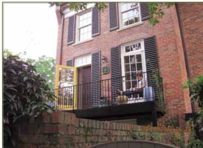
Soon enough, plans were completed, permits received, scheduling settled, and Cruickshank Remodeling began construction. The two double-hung windows with transoms were removed, the brick wall was cut and removed to the floor, and French doors with transoms were fit into the new openings. Custom shutters, longer than the originals, were installed flanking both doors to give it the final finishing touch.
